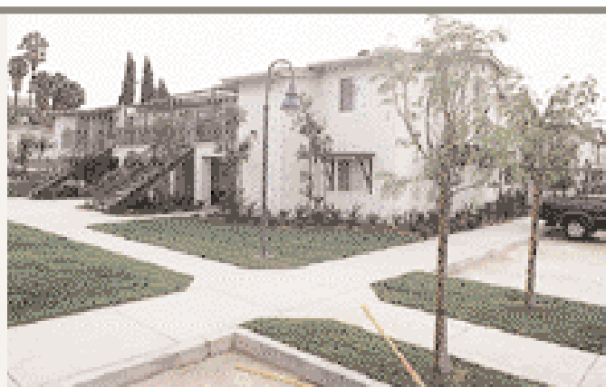
The rebuilt core of Jeffrey-Lynn is aesthetically pleasing and safer. By improving common-area lighting and replacing the narrow, crooked alleys and pathways with clear sight lines, crime has been reduced, making residents feel more secure.
